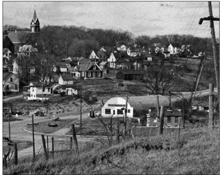
John Boyd built the Quonset hut at 411 Commerce St. to house his J. I. Case farm equipment dealership. The sign on the building says "Boyd Motors"; two gas pumps are visible in the front.
