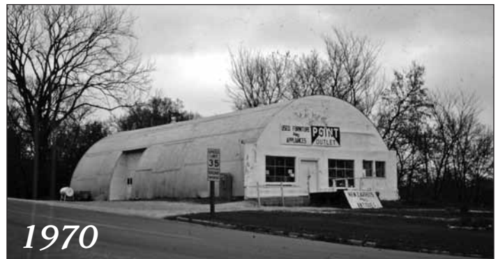
In 1970 the building housed Point Outlet, selling used furniture and appliances, new carpets, and antiques. The gas pumps have been removed.
