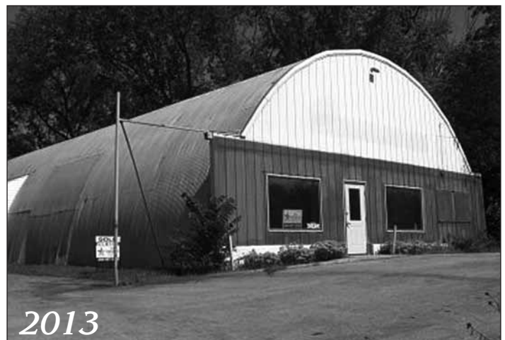
The location of NAPA Auto parts for many years, the Quonset hut was sold earlier this year to Shake Rag Alley and will be renovated and used by the arts school for classrooms.
