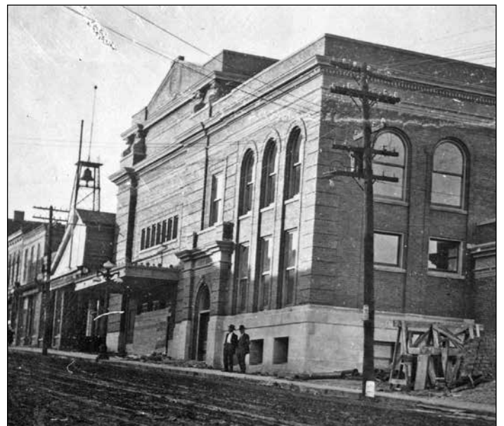
Even when the Municipal Building was almost ready for occupancy, half of the building next door, the former county office, was still standing.
