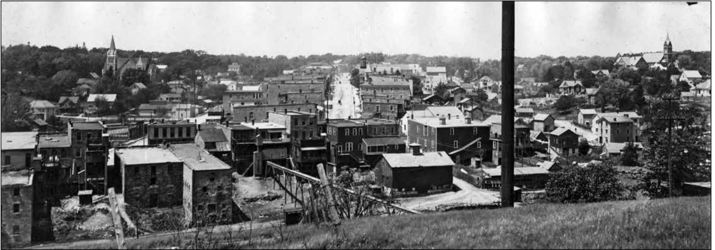
View down High Street from the power station site, before erection of the concrete chimney.
