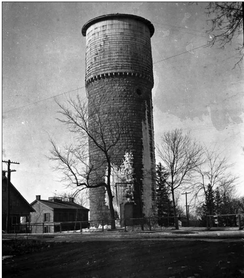
The original water tower was built of brick and wood and served the community from 1898 until 1916. Before this, water was supplied to home and business by private wells in the backyard, cisterns and rain barrels, and the hand-pumps at Jerusalem Spring on Fountain street and Federal Spring on Shake Rag street.
